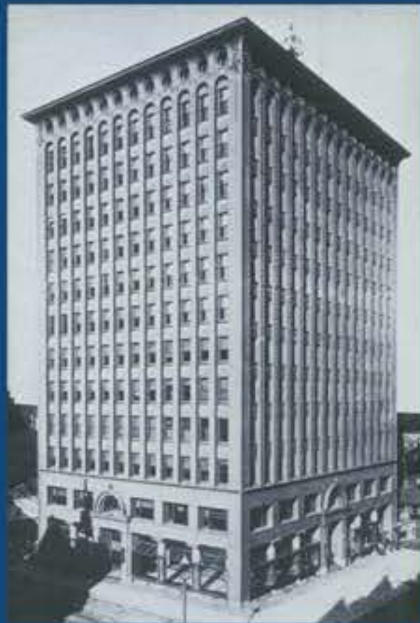
Guaranty Building, Buffalo, USA, 1896
